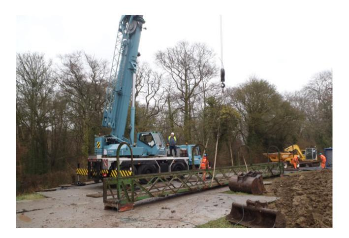
A retrofitted bracing arch, fabricated to match the existing brace arches, was checked for alignment and match drilled with the existing bridge before disassembly. The new steel angle for fixing to the abutments was also checked for alignment with the existing bridge components, and templated before disassembly.
